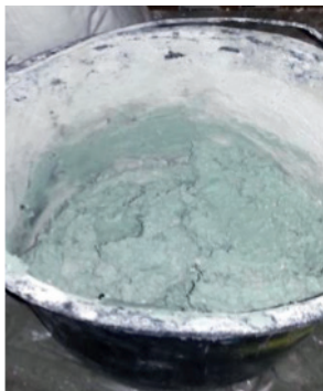
Mix GPG Marine to desired consistency
